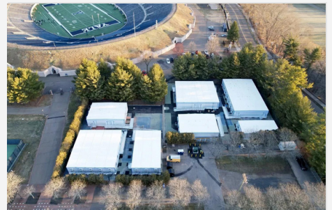
Custom Locker Rooms For Yale University
